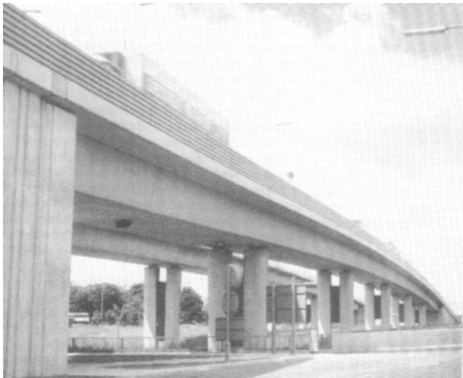
Fig 1.8 - Un pont à tablier continu [tiré de Pritchard B. 1992 Bridge design for economy and durability , Thomas Telford Services London, 172 p.].
